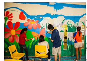
Some JCU Singapore staff are painting the walls of a welfare centre in Singapore.
